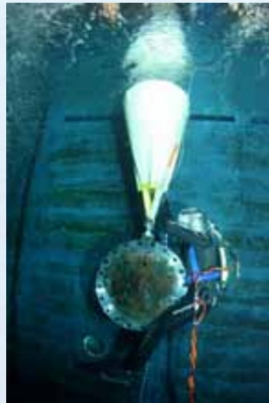
Commercial Lift Bag replacing a flange plate at the Atlanta Aquarium.
