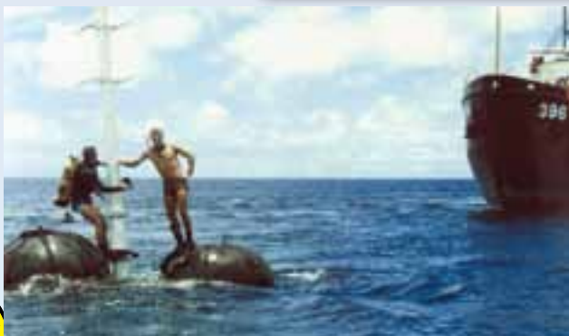
US Coastguard Divers using Professional Lift Bags to lift and service a communication and monitoring tower.
